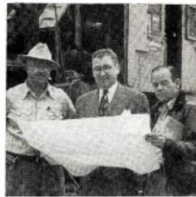
CONSTRUCTION has started on the new KCBS San Francisco 50 kw transmitter in Novato, Calif. Discussing progress at the Marin County site are (l to r) Charles Hageman, construction crew foreman; Arthur Hull Hayes, vice president for CBS in San Francisco and general manager of KCBS, and Alan Cormack, chief engineer of KCBS.
